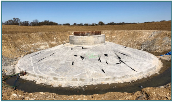
Completed base of wind turbine
