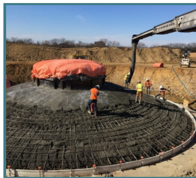
Pouring base of wind turbine
