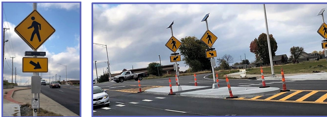
New RRFB pedestrian crossing installed on 20 th Street, Joplin, MO
