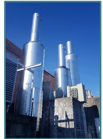
CWEP new exhaust stacks housing catalytic converters
